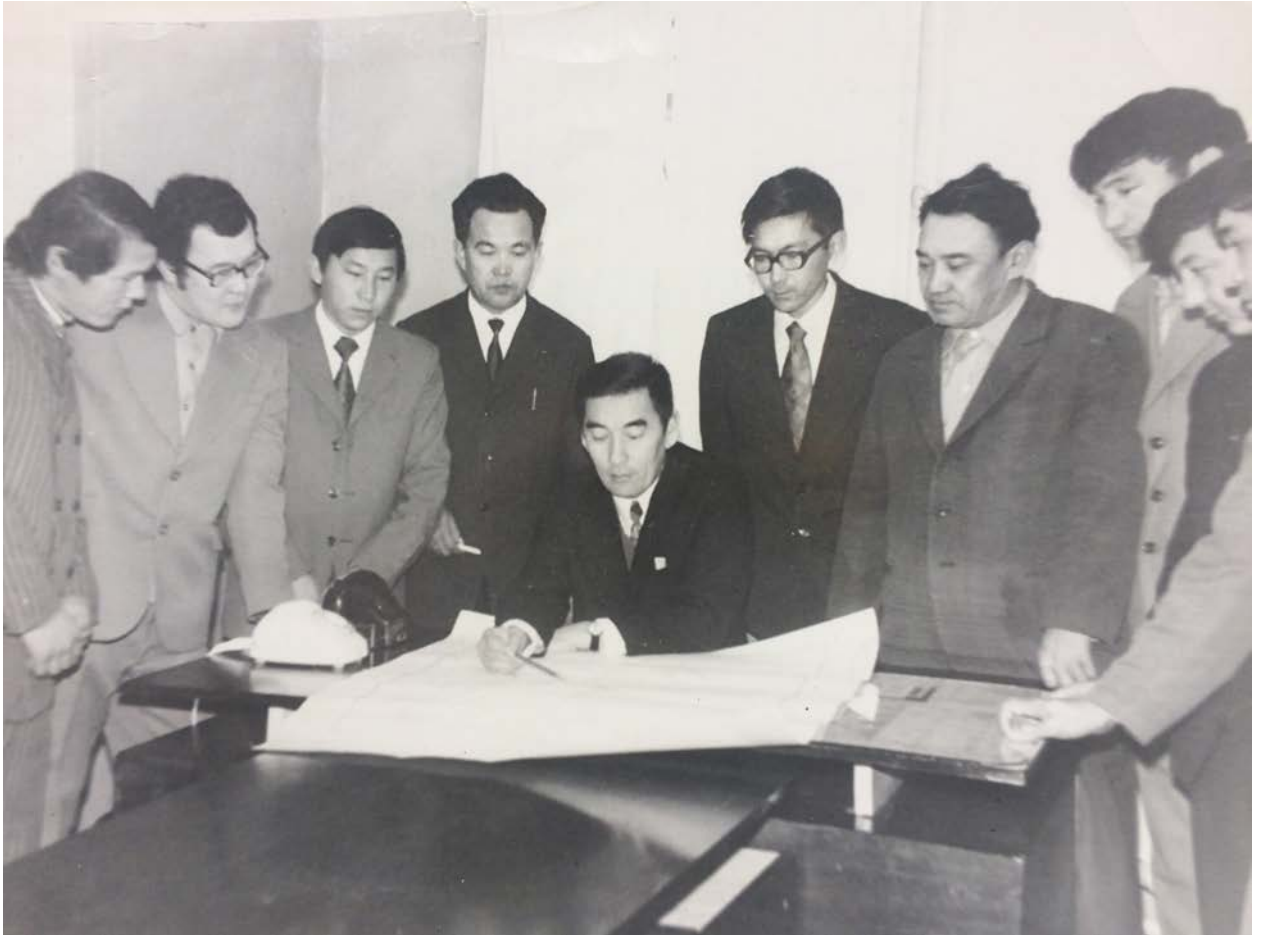
New exploration zone being discussed
